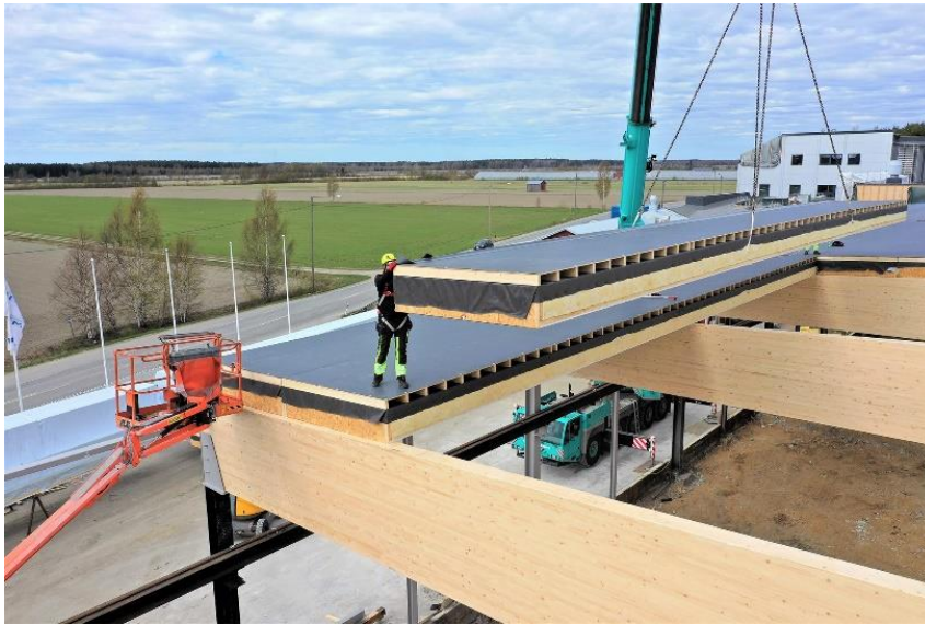
Figure 19. Roof elements can be installed quickly. Photo: www.termater.fi
