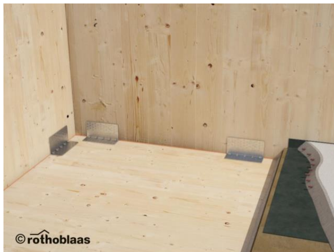
Figure 8. Example of fastening solid wood panels from Pauli Paintola’s presentation at the Puurakentaminen – kiinnikkeet ja liittimet event held on 29 October 2019 in Ähtäri. The figure features Rothoblaas fasteners.
