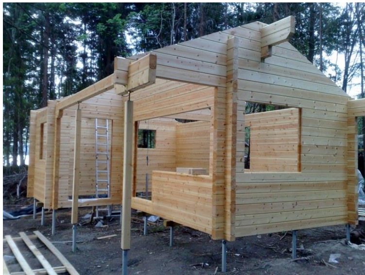
Figure 23. Log frame erected on a screw pile foundation. Photo: www.paalupiste.com
