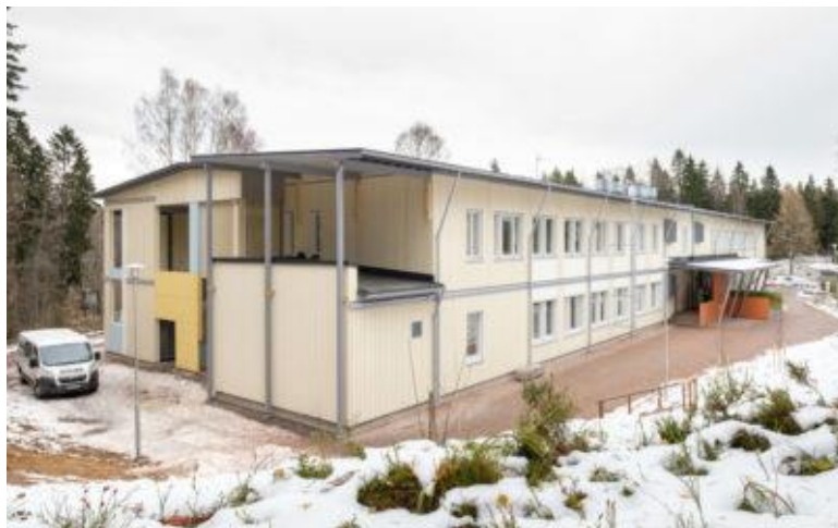
Figure 2. A portable two-storey school building constructed by Parmaco Oy and located in Espoo. The school meets the requirements of new learning environments: the spaces are open, modifiable and contain learning areas of different sizes for varying needs. Photo: www.parmaco.fi
