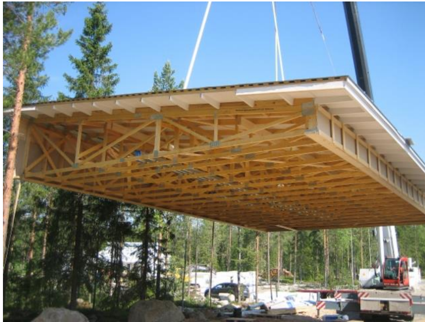
Figure 18. Lifting a roof element onto a detached house. Photo: www.abc-service.fi
