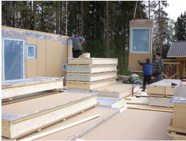
Figure 14. Erecting small elements. Photo: Harri Lyytinen, 2012.
