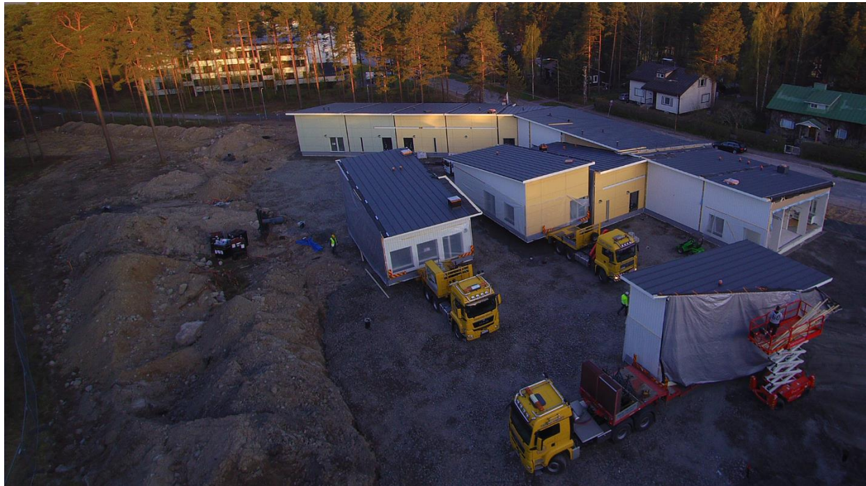
Figure 22. Installing Teijo-Talot modules on a gravel bed. (Teijo-Talot presentation in Seinäjoki on 9 May 2019)
