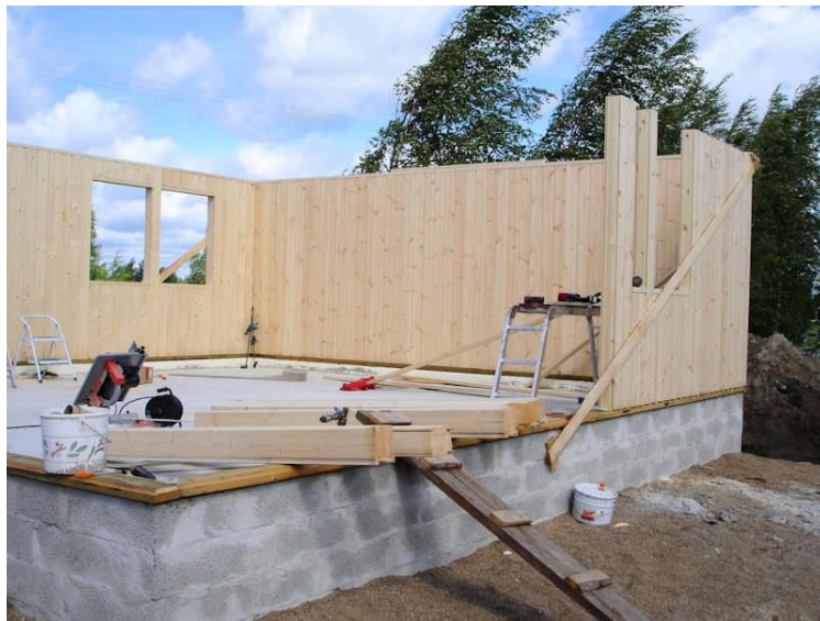
Figure 13. When erected on site, it can be assembled by a single person since the logs are light and easy to handle thanks to their dimensions. Photo: www.pystyhirsi.fi
