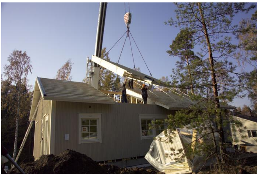
Figure 20. Installing a roof face element. Photo: www.simons.fi
