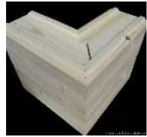
Figure 37. Mitred corner joints (Pluspuu, 2017d)
