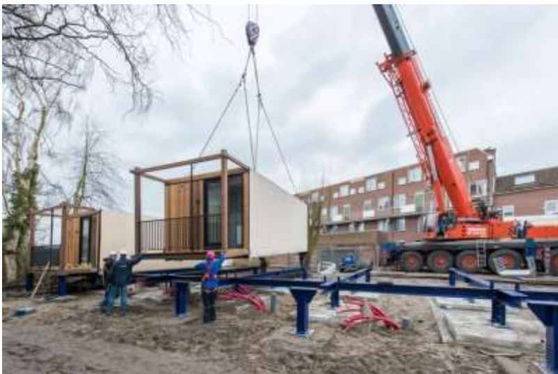
Figure 25. Placement of the module (Finch Buildings, 2017)
