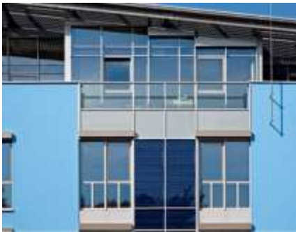
Figure 89. Solar modules (Schüco, 2017)
