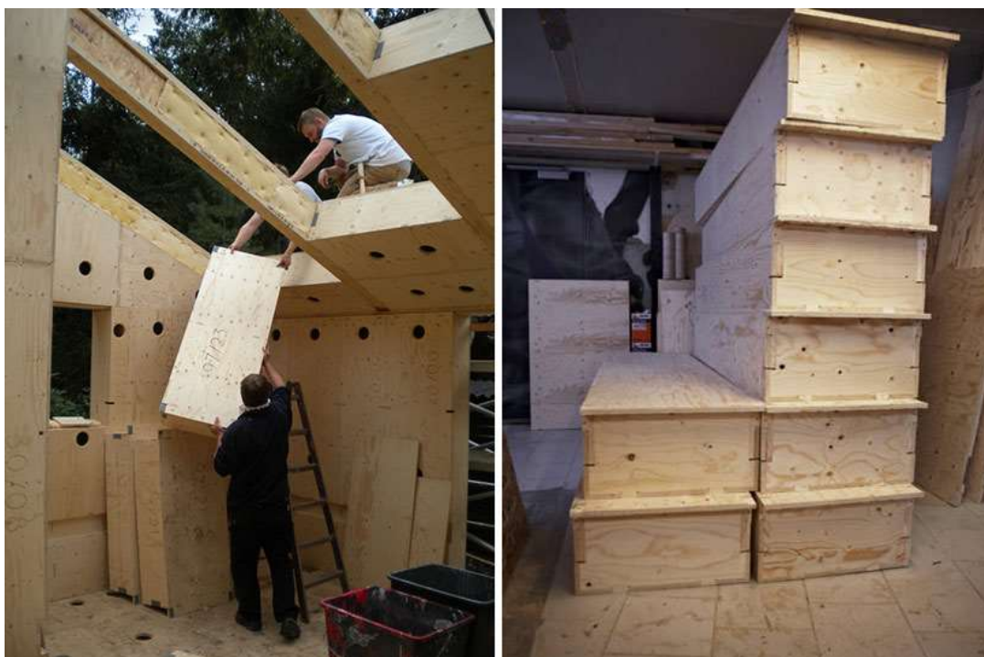
Figure 41. Modular segments and building process (Eentileen, 2012)
