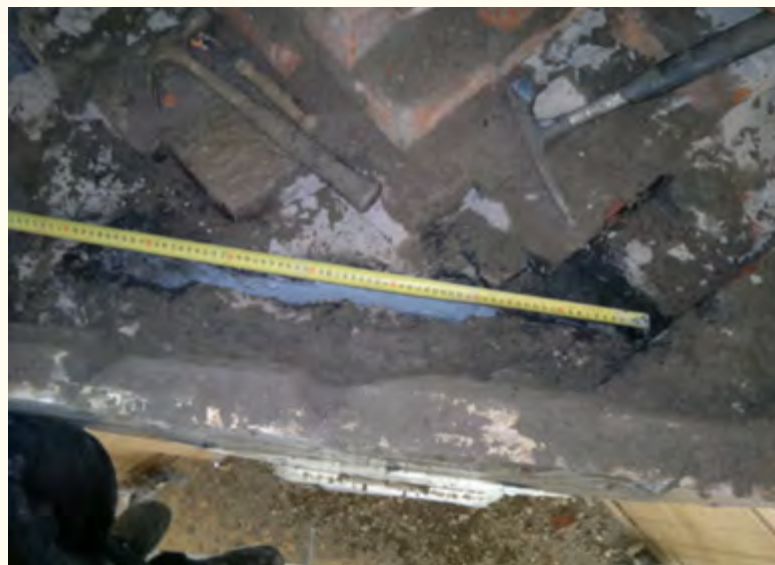
Figures 2.8 a, b. The smoke flue becomes visible two bricks down from the top of the fourth tile row. Above: measured drawing of the same.
