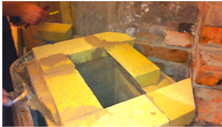
Figure 1.24. Installing the second row of sawn bricks.
