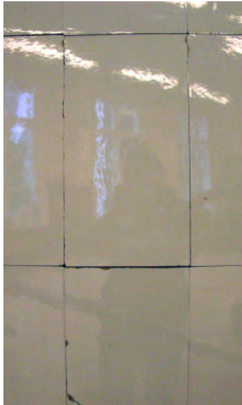
Figure 1.49. The face of the stove before joints and cracks were filled.
