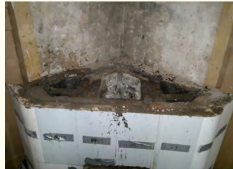
Figures 2.13 a, b. Top view of the ninth row of tiles. Here we can see the top of the furnace. Above: measured drawing of the same.
