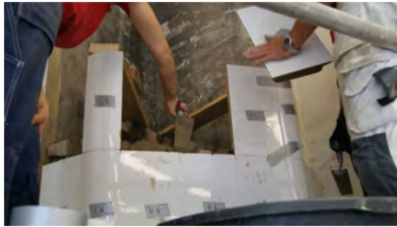
Figure 1.29. Installing the middle tiles on a bed of mortar.
