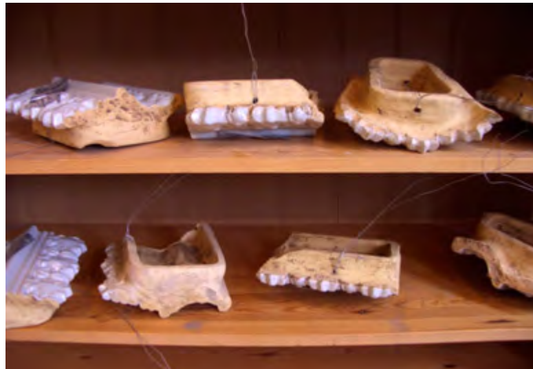
Figure 2.58. Crown tiles waiting to be installed.
