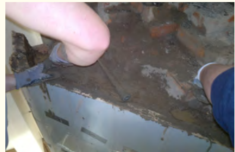
Figures 2.7 a, b. Top view of the fourth row of tiles. The brick work is still solid, i.e. none of the smoke flues that we were looking for are visible yet. Above: measured drawing of the same.
