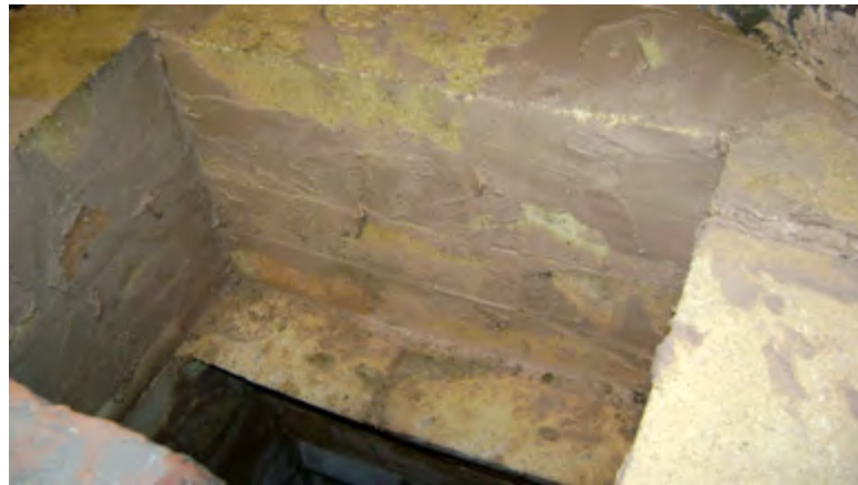
Figure 2.46. The bottle neck forms a shelf above the furnace.
