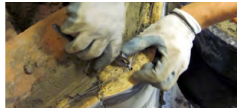
Figure 2.45. The baling wire is attached to the new nails.
