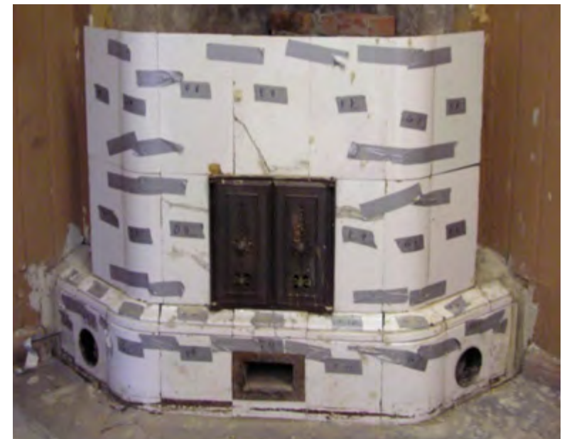
Figure 1.36. End of day 1. We had built our first row of tiles and the furnace behind it.
