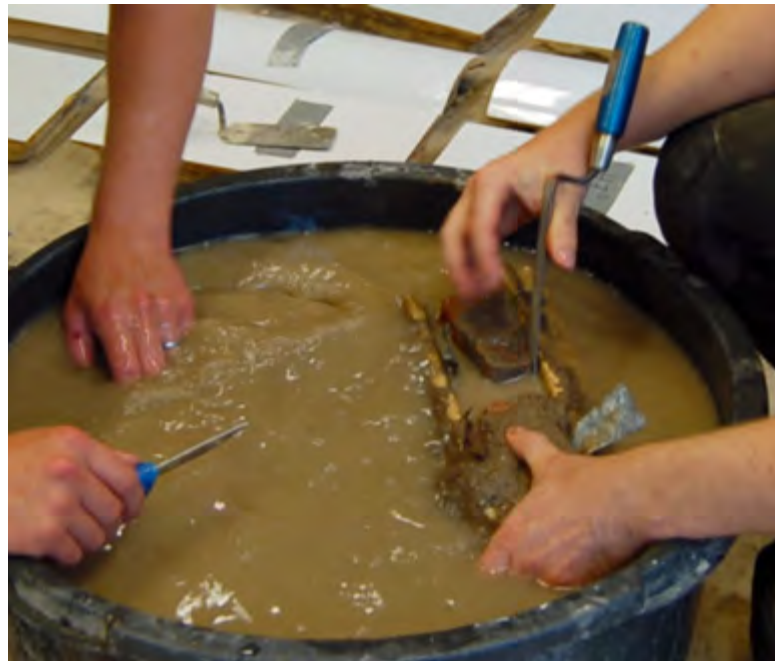
Figure 2.18. The bricks, the metal clamps and mortar on the backside of the tiles are being removed. This takes time and you have to be patient because the edges and corners chip easily. Traditionally also the metal parts were reused but we ran out of time for that.
