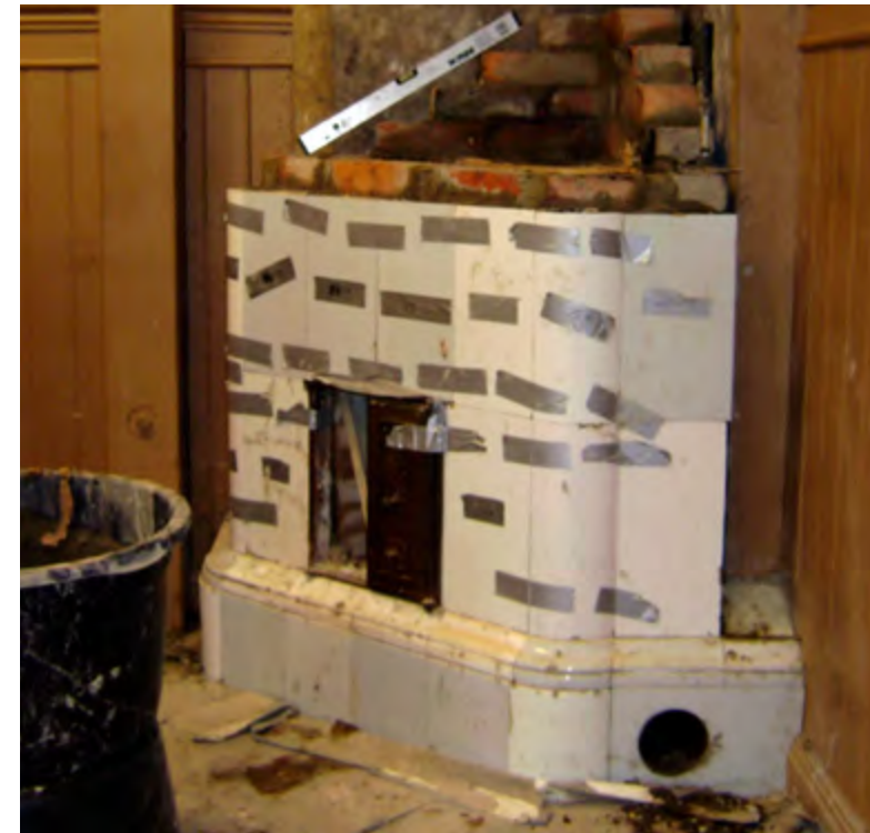
Figure 2.44. The rear brick wall and the front course is laid.
