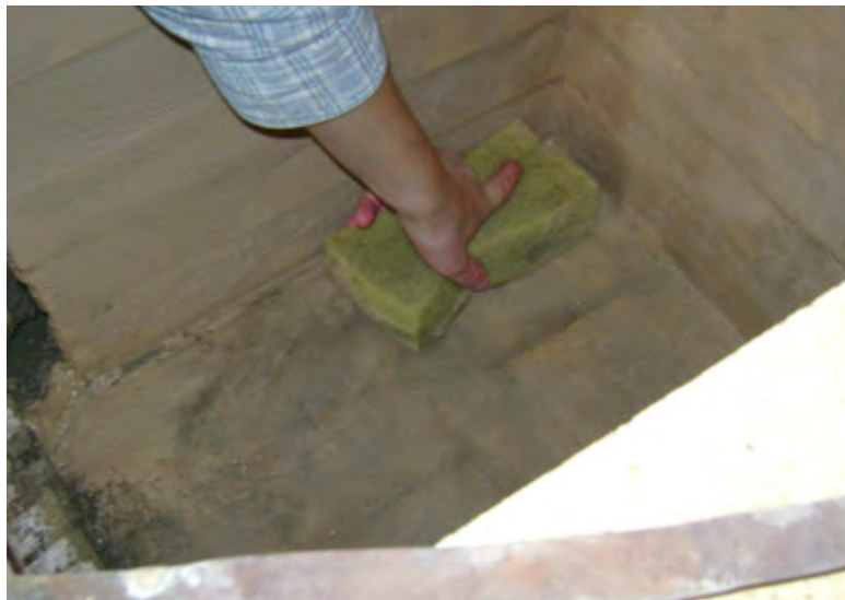
Figure 2.33. The bricks and joints are being washed with a moist sponge.
