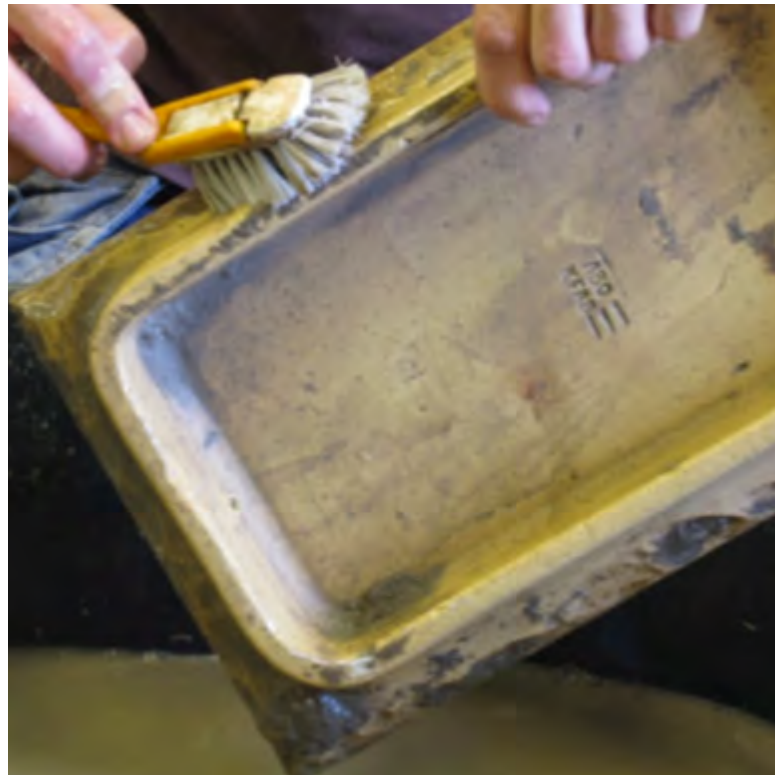
Figure 1.13. Brushing off remaining particles of mortar. The manufacturer's stamp, ÅBO KFAB, stands for Åbo Kakelfabrik Ab, the Swedish for Turun Kaakelitehdas Oy.
