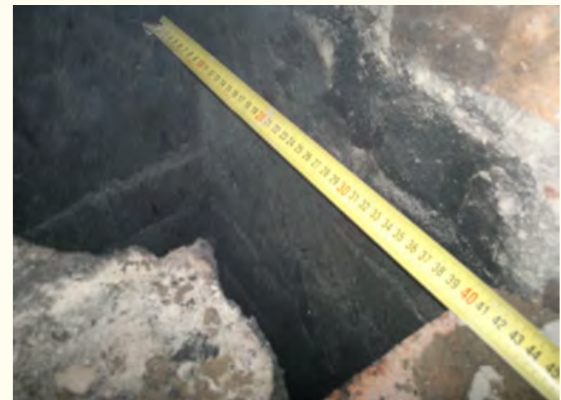
Figures 2.9 a, b. The rear smoke flue which leads to the chimney is found at the top of the fifth tile row. Above: drawing of the same.
