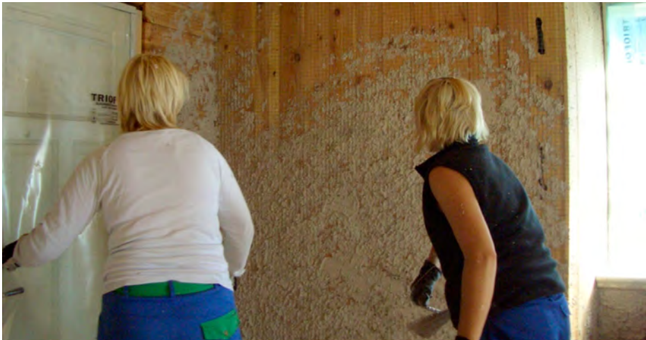
Figure 17. Making the plaster attach to wire netting was hard work.
