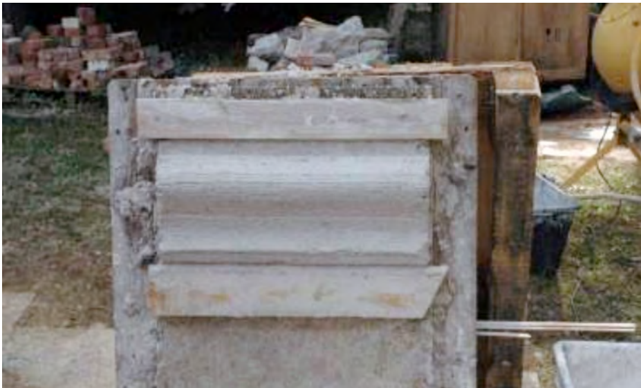
Figure 15. Moulding the surface by using a stencil.
