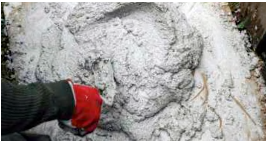
Figure 10. Mixing hot lime by hand.
