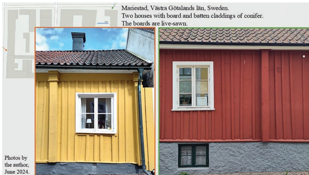
Figure 23: Board and batten claddings in Mariestad – Sweden.
