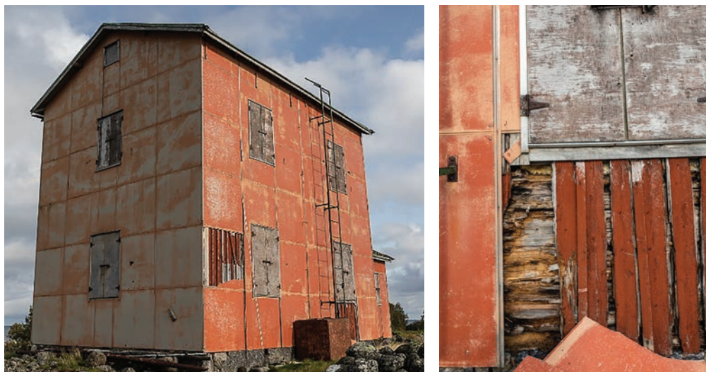
Figures 8 and 9. Ritgrund main building, pilot station. To the right detail of rotten structure behind the plates. Photo: Author.
