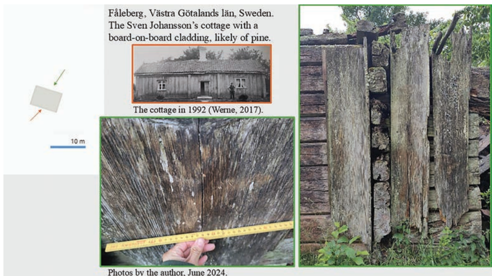
Figure 11: Board-on-board cladding in Fåleberg – Sweden.
