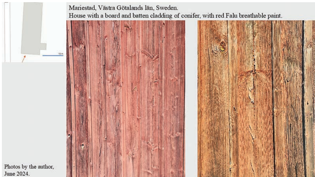
Figure 18: Board and batten cladding in Mariestad – Sweden.
