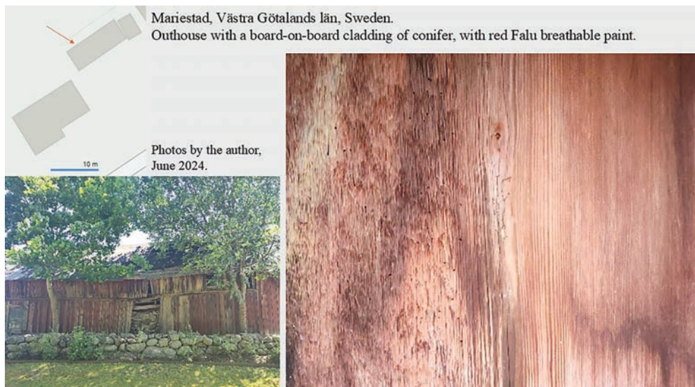
Figure 22: Board-on-board cladding in Mariestad – Sweden.
