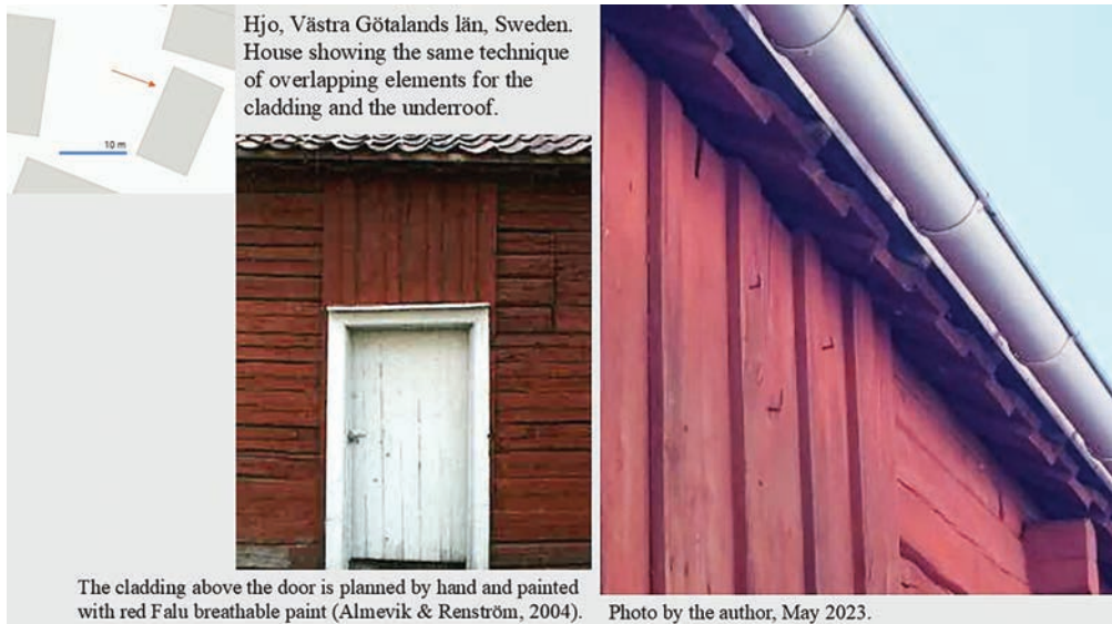
Figure 17: Lapped elements in Hjo – Sweden.
