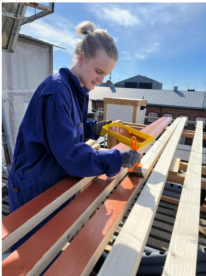
Figure 48: Painting of the wooden beams
