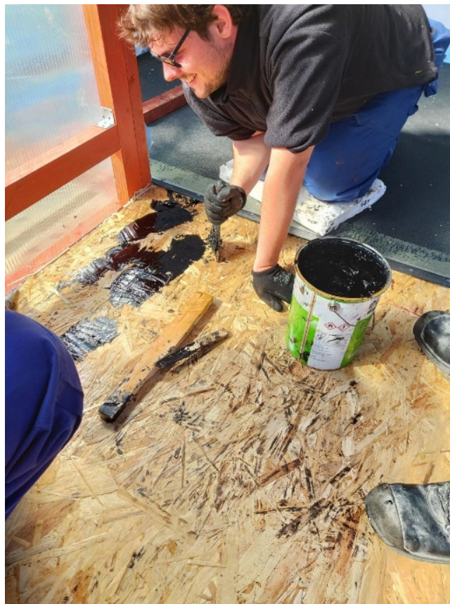
Figure 55: Spreading glue for the tarred roof paper on the OSB plates
