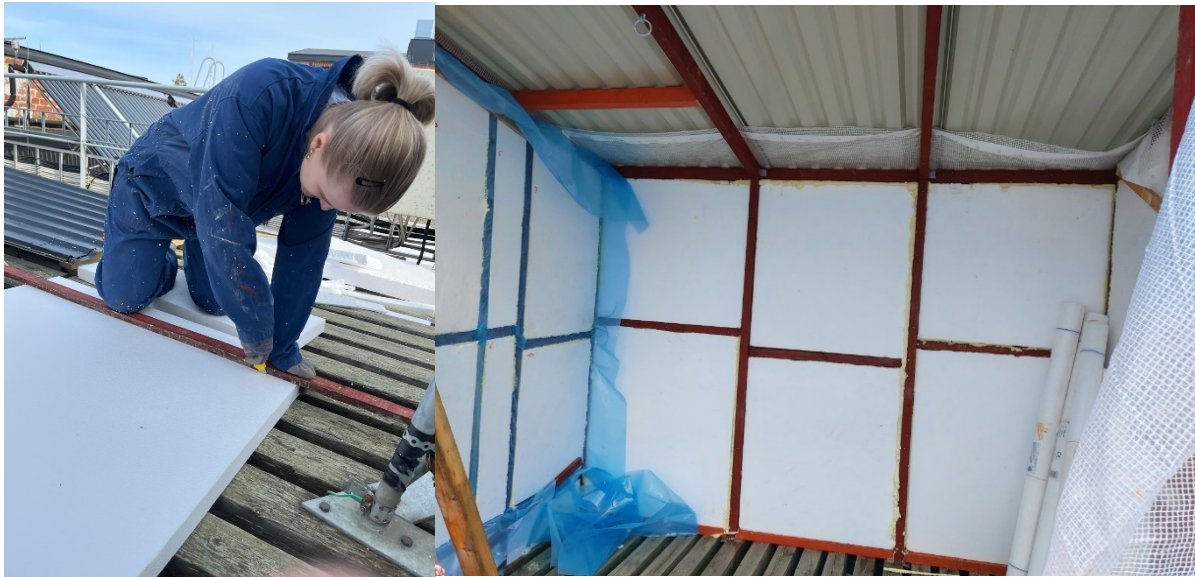
Figure 51: Cutting EPS
