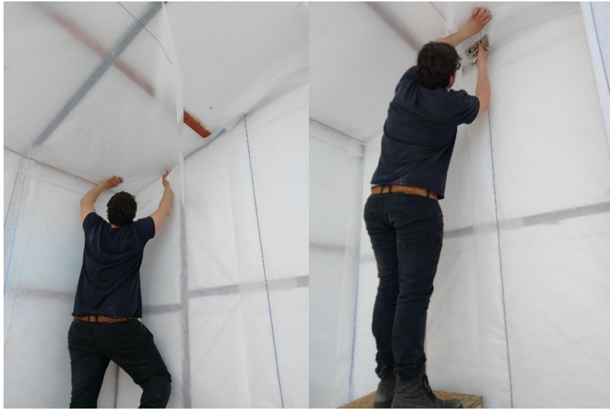
Figure 57: Attaching of the white foil
