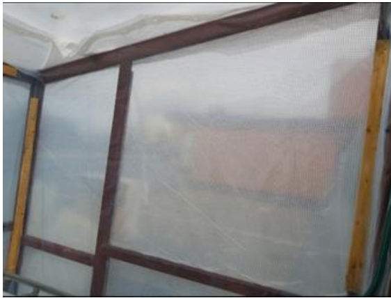
Figure 77. Example of the reinforcements to the inside isolation.
