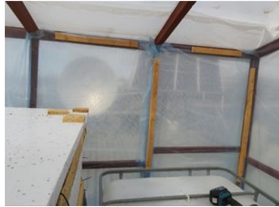
Figure 77. Example of the reinforcements to the inside isolation.
