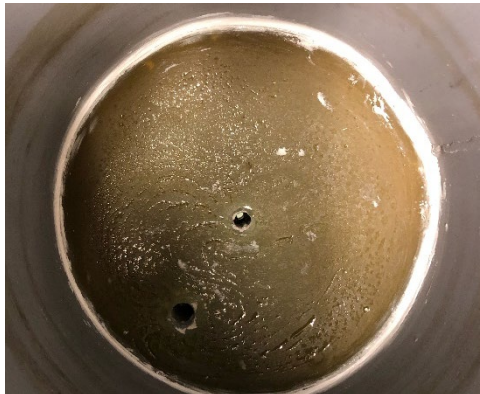
Figure 50 Gaps filled up with polyester
