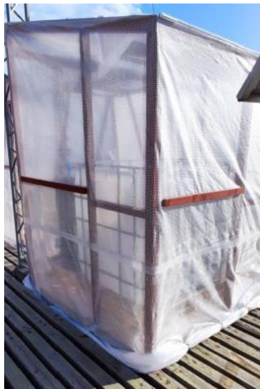
Figure 5: Repairing the walls, view of the previous PE foil installed
