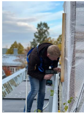
Figure 8: Repairing the walls, attaching the PE foil
