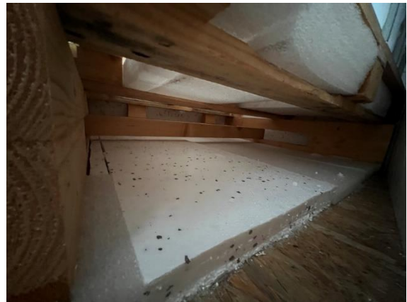
Figure 32: Insulation of the bottom of the main tank
