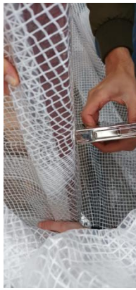
Figure 8: Repairing the walls, attaching the PE foil
