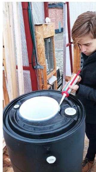
Figure 34: Team member applying silicone to the sedimentation tank
