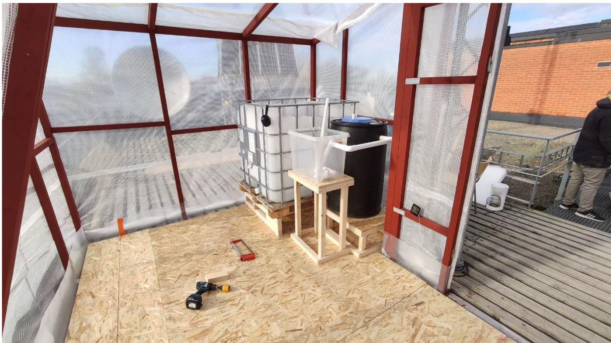
Figure 4.19 Covering the floor with wooden chipboard
