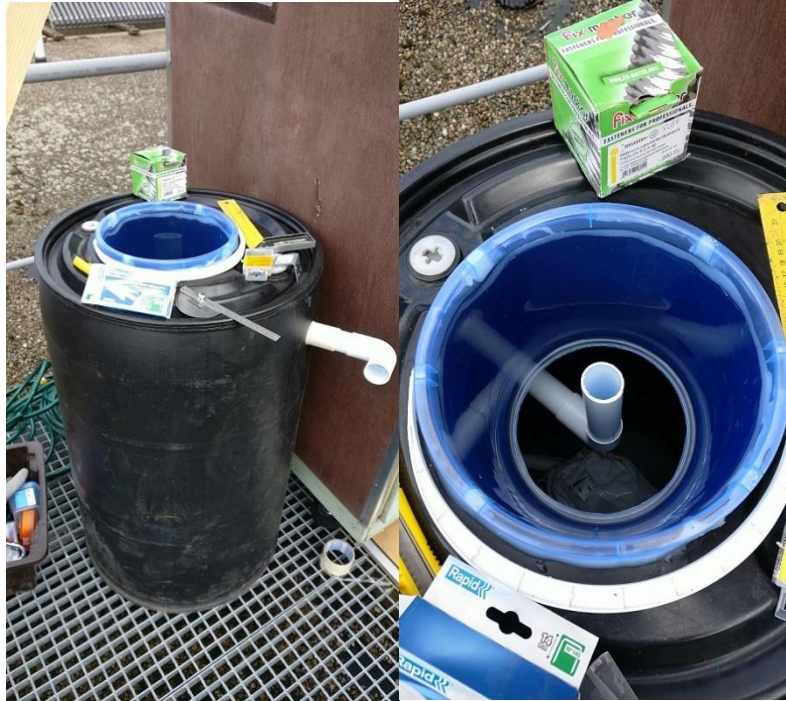
Figure 2.44 Settling tank building process
