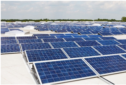
Figure 22: Solar panels mounted on a flat roof
