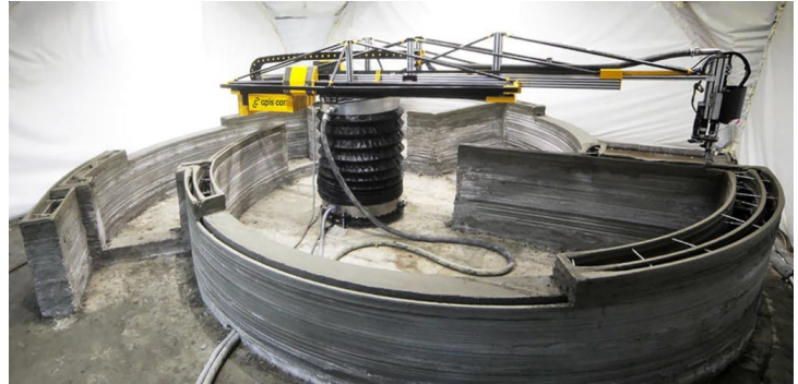
Figure 27: FDM printer printing a house (source: Apis cor)
