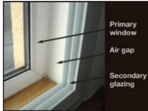
Figure 60 Secondary glazing system <sup>[33]</sup>
