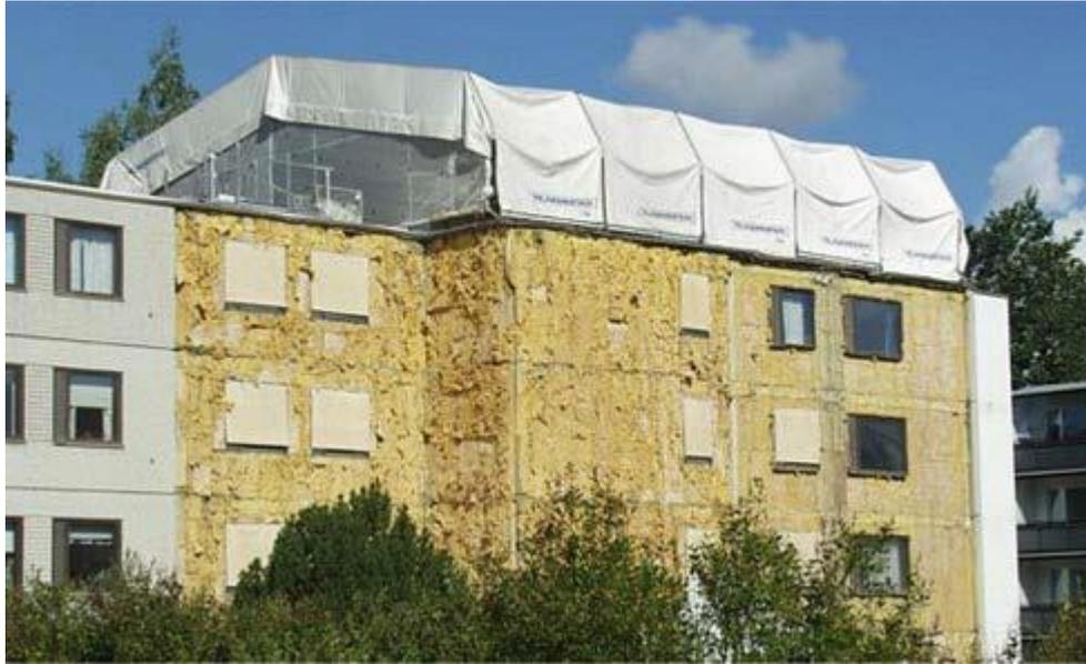
*Fig. 6 Demolition of old insulation and outer pane of facade*
