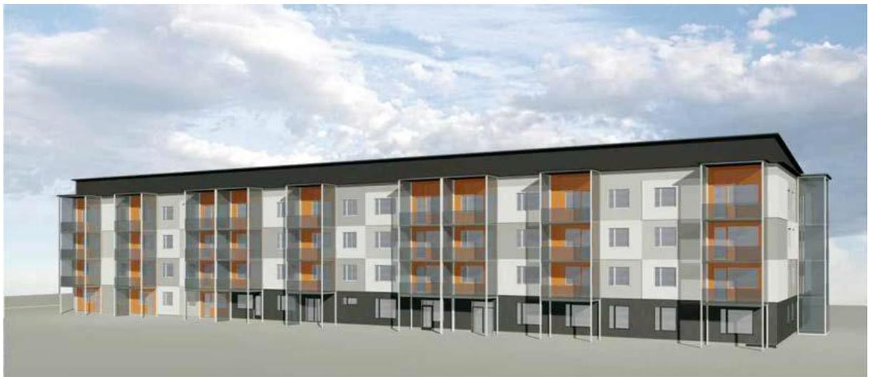
*Fig. 8 Building after full renovation with TES facade, new balconies and new tilted roof (source: arch. Kimmo Lylykangas)*
