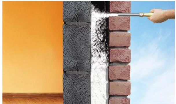
Figure 50 Cavity wall Insulation
