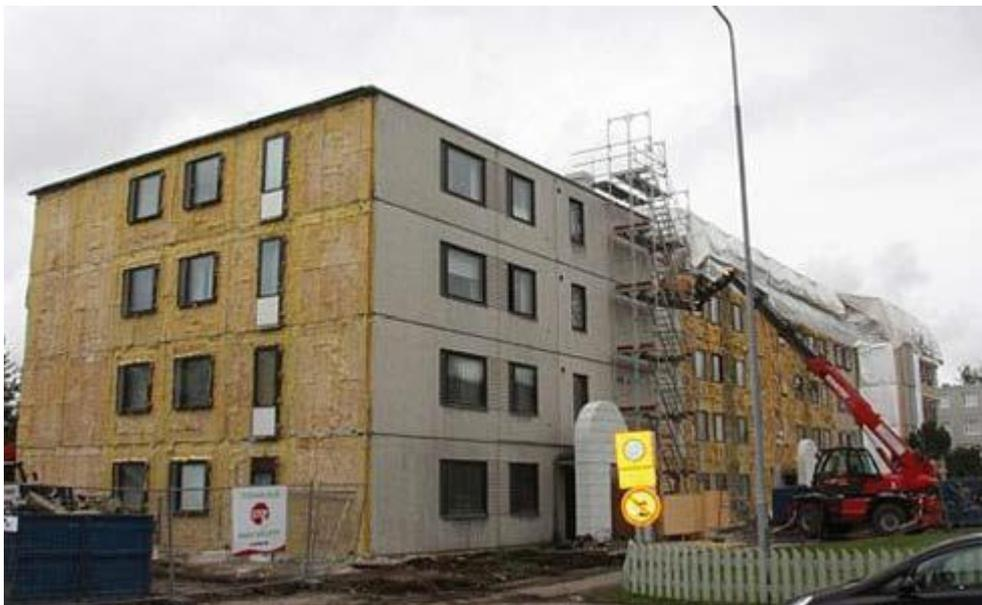
*Fig. 5 Demolition of old insulation and outer pane of facade*
