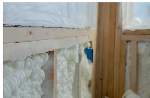
Figure 52 Cavity wall insulation
