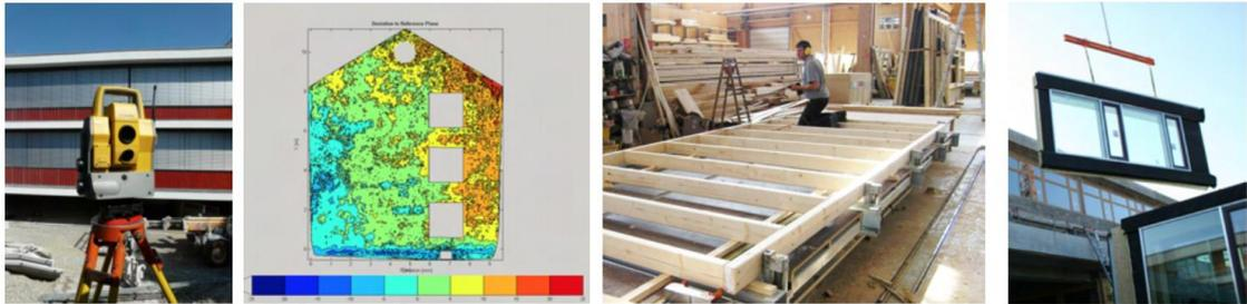
Figure 54 TES method; From survey to assembly <sup>[16]</sup>
