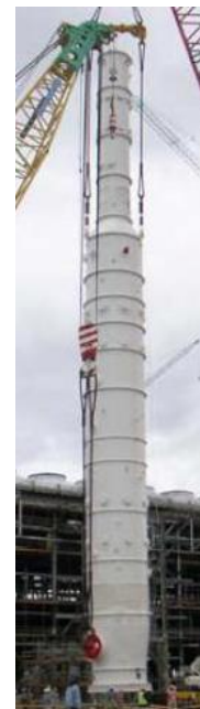
Figure 14 Cryogenic heat exchanger tower used for liquefaction of natural gas
