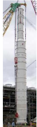
Figure 91: Cryogenic heat exchanger tower used for liquefaction of natural gas
