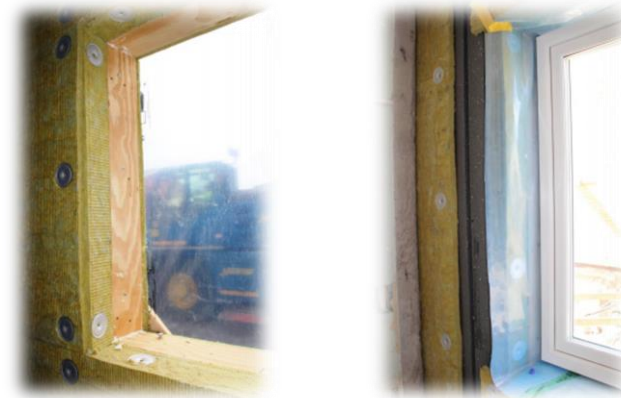
Figure 82: New windows installation.
