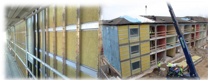
Figure 77: Insulation installation.
