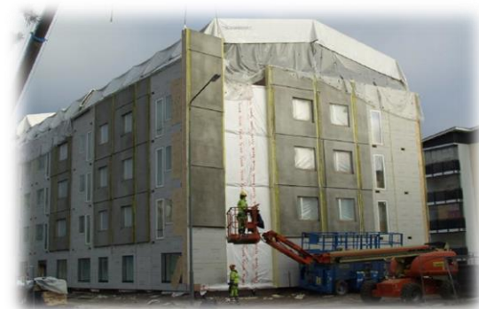
Figure 66: Installation of the facade 2.
