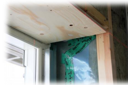
Figure 84: New window insulation.
