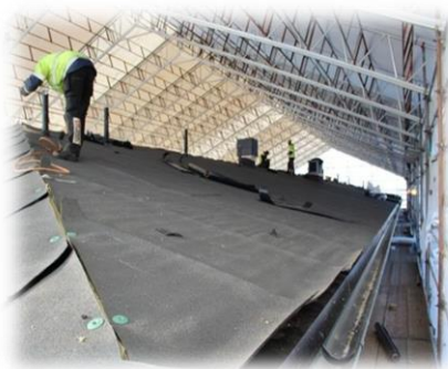
Figure 80: Insulation roof renovation.
