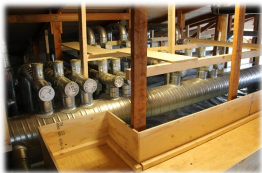
Figure 83: Installation steps of the insulation attic.
