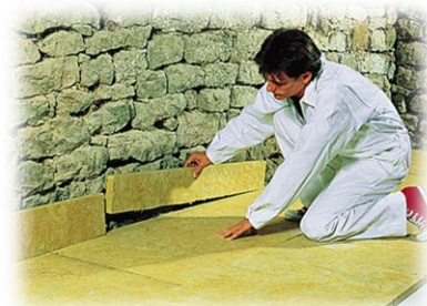
Figure 34: Supple insulation. Maisonbrico .com 2016
