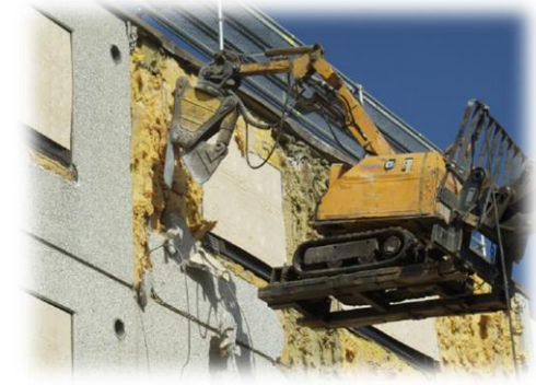
Figure 62: Case 1. Demolition of facade.
