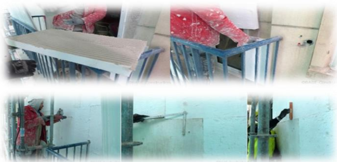
Figure 97: BASF MultiTherm aero installation
