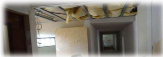
Figure 98: Acoustic insulation in common areas.
