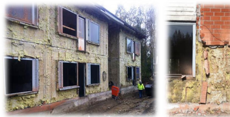
Figure 70: Removal of facade.
