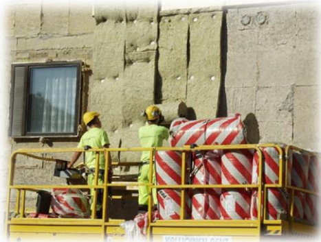
Figure 64: New insulation installation.
