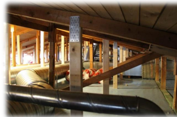
Figure 81: Heating ducts location.
