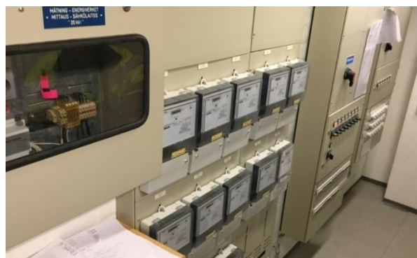
Figure 23 Meters of electricity consumption
