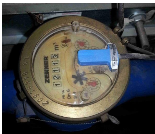
Figure 6: Left side: Water meter with (blue) reed contact switch for pulse output on top of it. Right side: Connection terminal next to the electricity meter (original state), where the pulse output was connected by the technician to the already existing telephone/signal cable.
