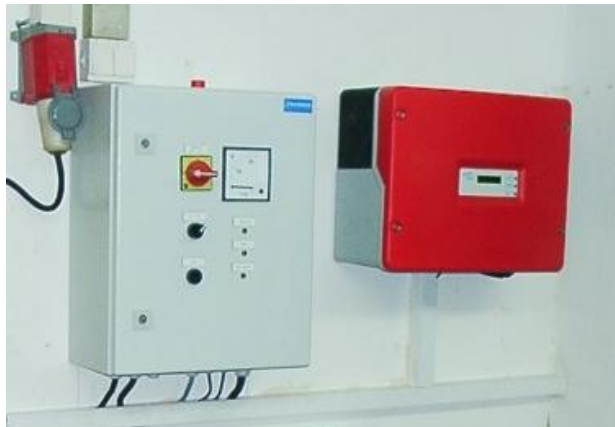
4.F. 11: Electrical housing and inverter
