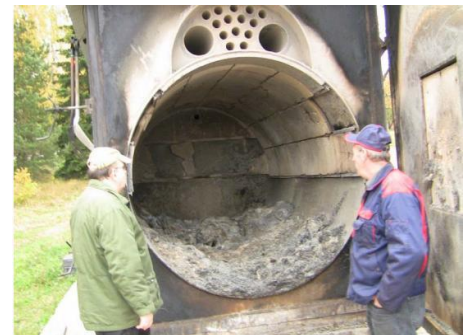
6.F. 14: Inside of a large biomass boiler
